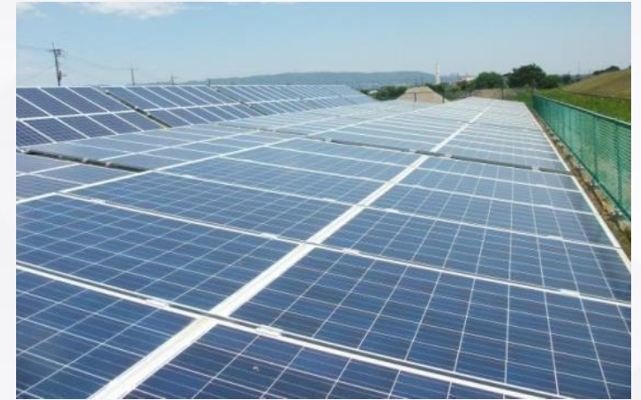
25 MW 2015-2016 in Tinglev , Denmark
